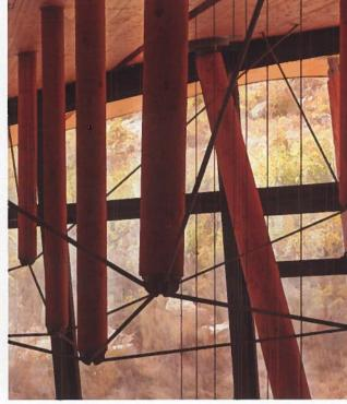
the roof are straight. The undulating surface is capped with several layers of plywood to create rigidity in the direction perpendicular to the lumber. The orthotropic nature of the wood plate was considered in the structural analysis using finite element software.
