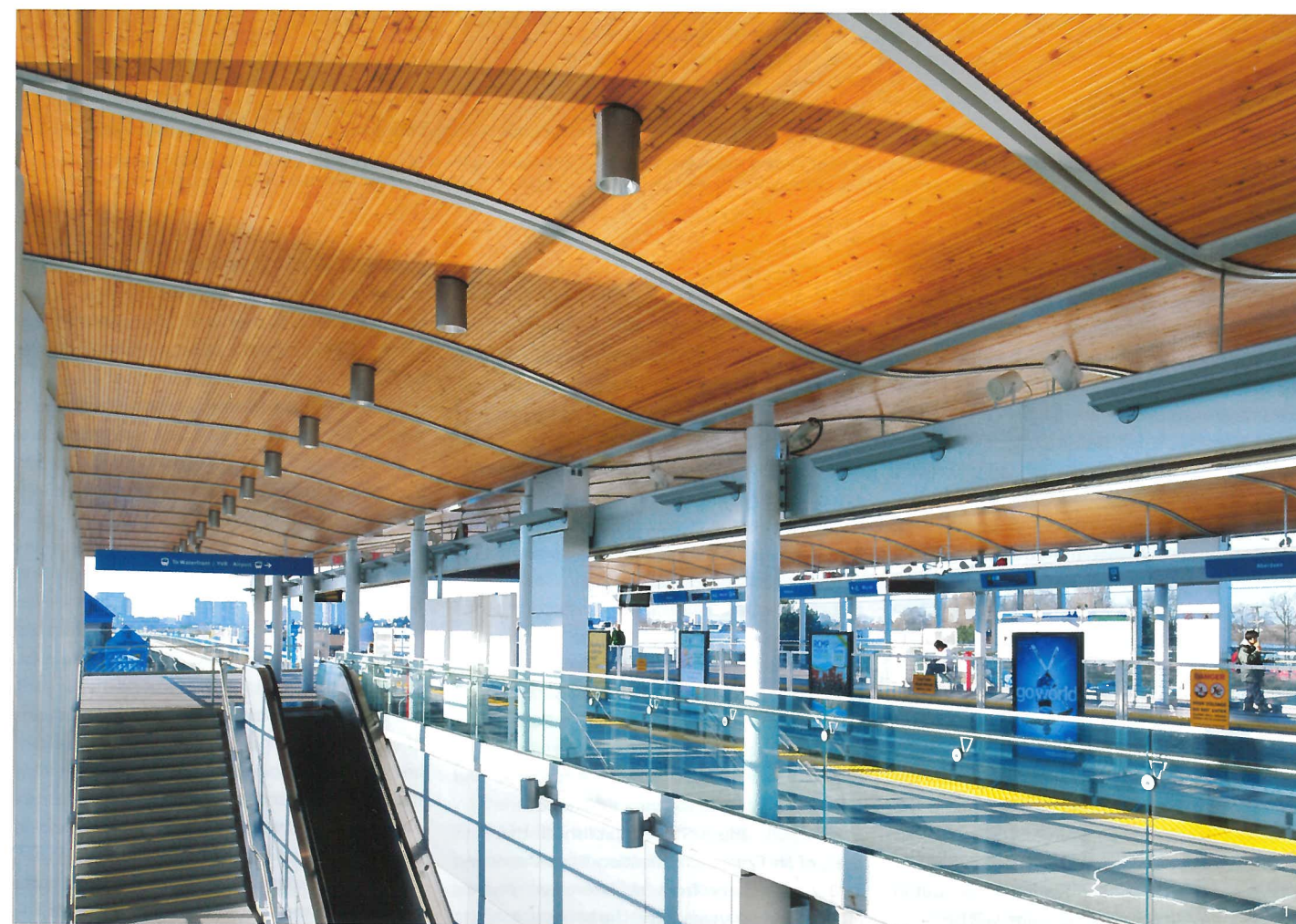
CANOPIES FOR THE CANADA LINE STATIONS WERE CONSTRUCTED USING MODULAR PREFABRICATED PANELS THAT INCORPORATE SOLID WOOD ELEMENTS WITHIN A STEEL CHANNEL FRAME. PHOTO: MARTIN TESSLER, COURTESY BUSBY PERKINS + WILL ARCHITECTS CO. [1].
