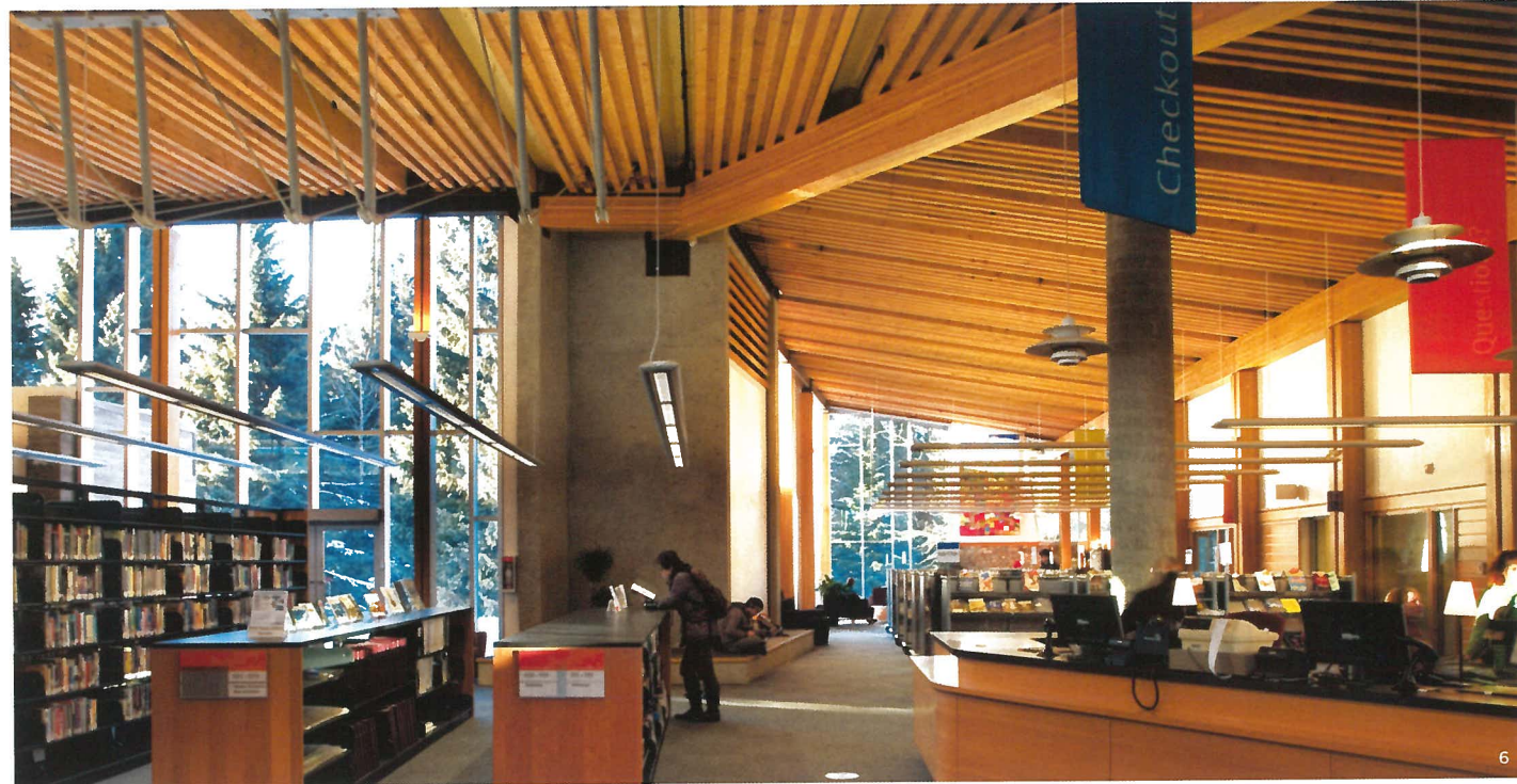
LOCALLY SOURCED AND FABRICATED HEMLOCK WAS USED FOR THE ROOF OF THE WHISTLER PUBLIC LIBRARY. PHOTO: NIC LEHOUX [6].
