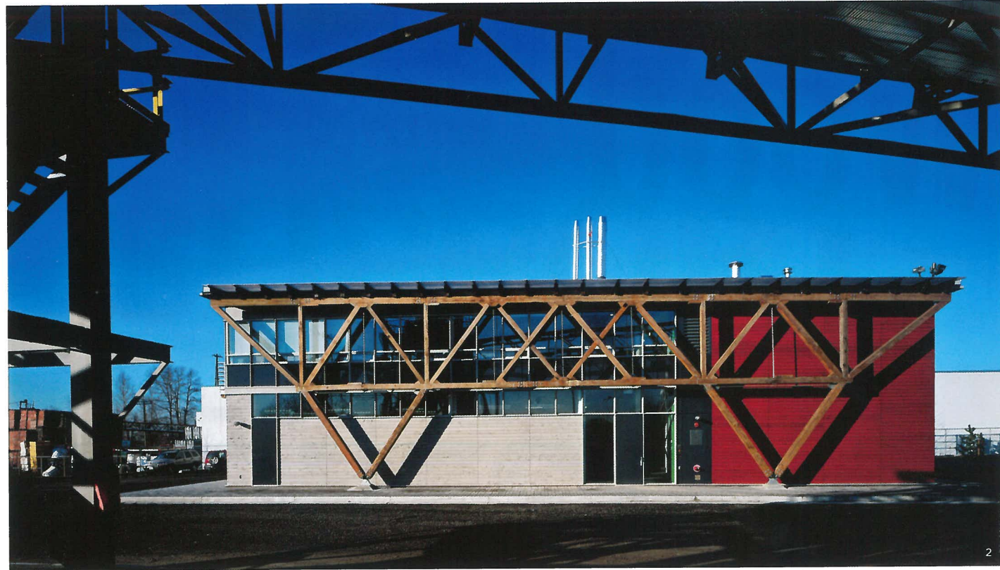
THE STRUCTURE FOR THE MATERIALS TESTING FACILITY INCLUDES MORE THAN 95% RECLAIMED WOOD. PHOTO: MARTIN TESSLER, COURTESY BUSBY PERKINS + WILL ARCHITECTS CO. [2].
