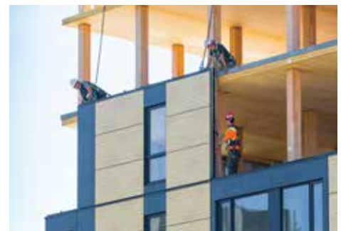
Figure 7. Perimeter envelope installation. Courtesy of Naturally: Wood and Steven Errico.
