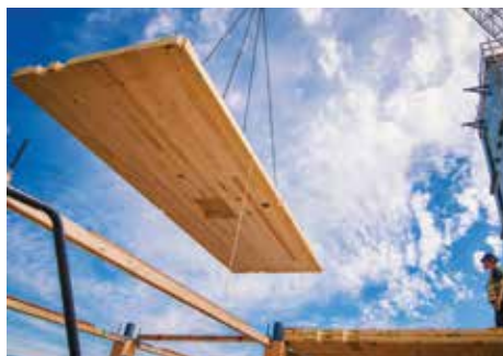
Figure 6. CLT panel installation. Courtesy of Seagate Structures and Pollux Chung.
