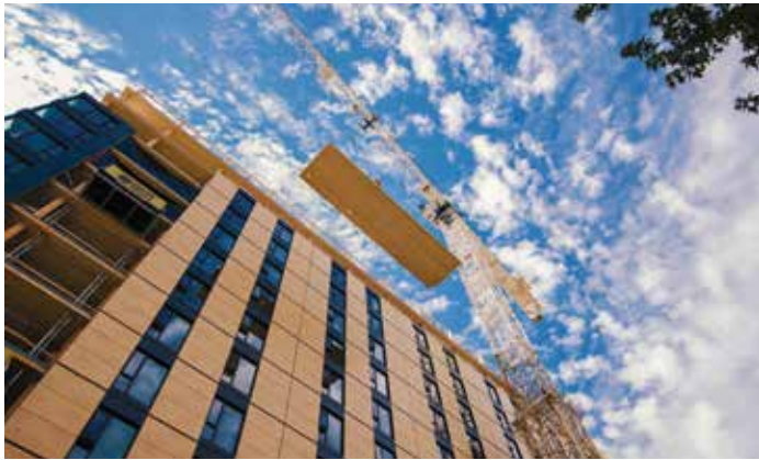
Figure 1. Timber erection – Summer 2016. Courtesy of Seagate Structures and Pollux Chung.
