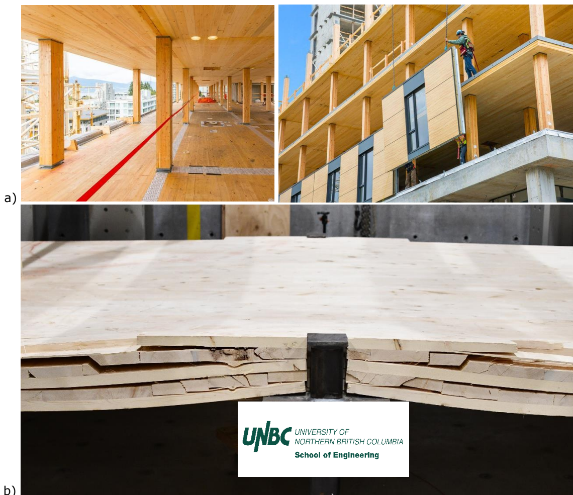
Figure 1: Point-supported CLT floor: a) UBC Tall-Wood house, photo credit: Fast+Epp; b) Punching shear failure, photo credit: Thomas Tannert
