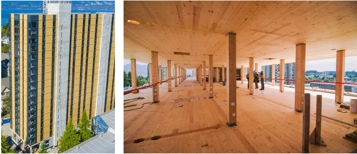
Figure 1. UBC Brock Commons (left); point supported floors (right) (Photos courtesy of Fast + Epp)
