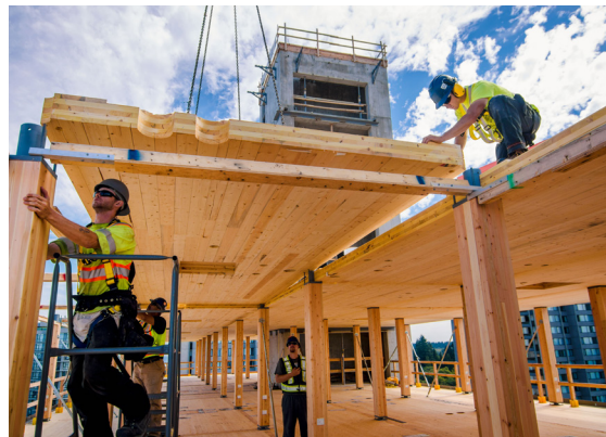
EMTC, Façade, Point-supported CLT, and Concrete
