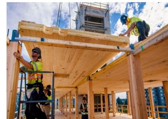
EMTC Facade, Point-supported CLT, and Concrete
