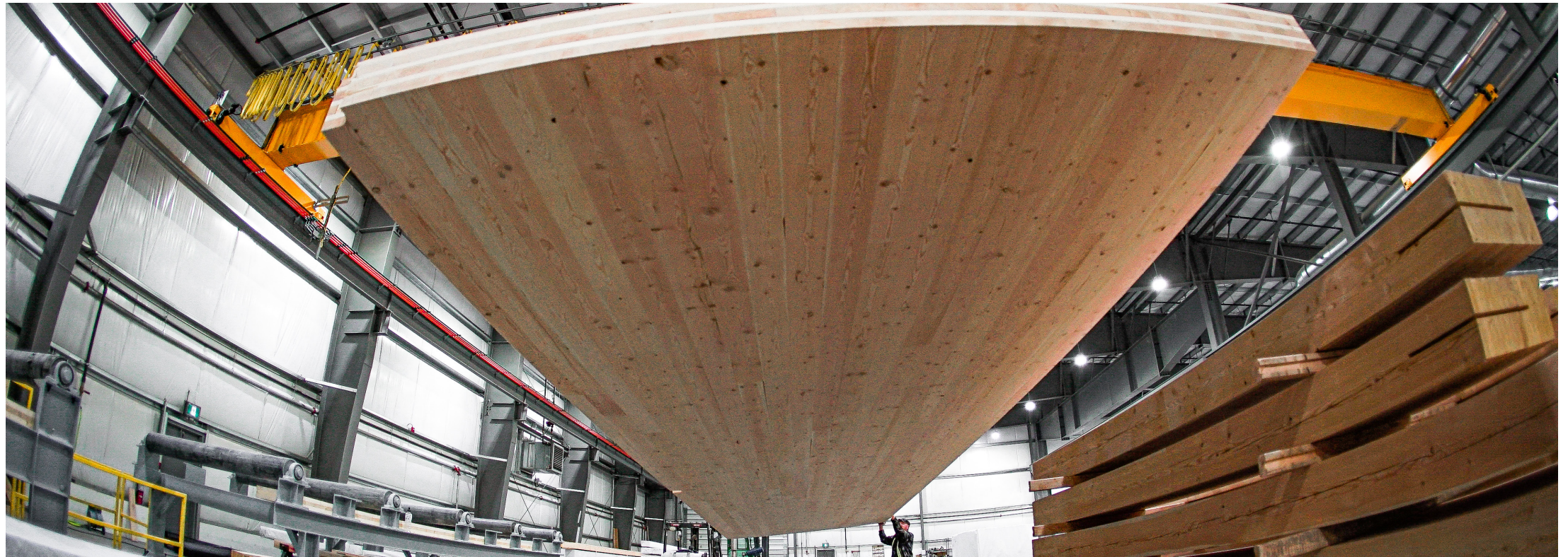
Photo of CLT CNC Fabrication. (Kalesnikoff)
