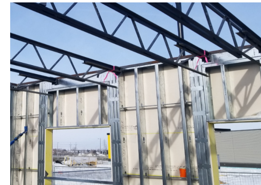
Steel stud, Steel Web Joists, and Concrete
