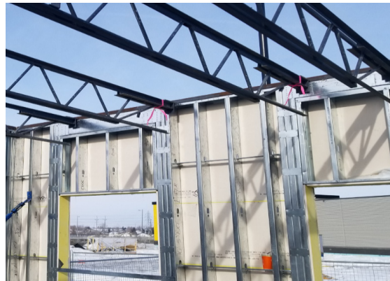
Steel stud, Steel Web Joists, and Concrete
