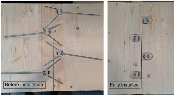
Fig 2: T-joint layout
