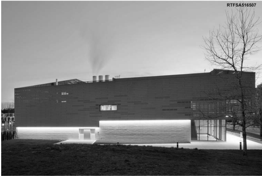
UBC District Energy Centre (4)
